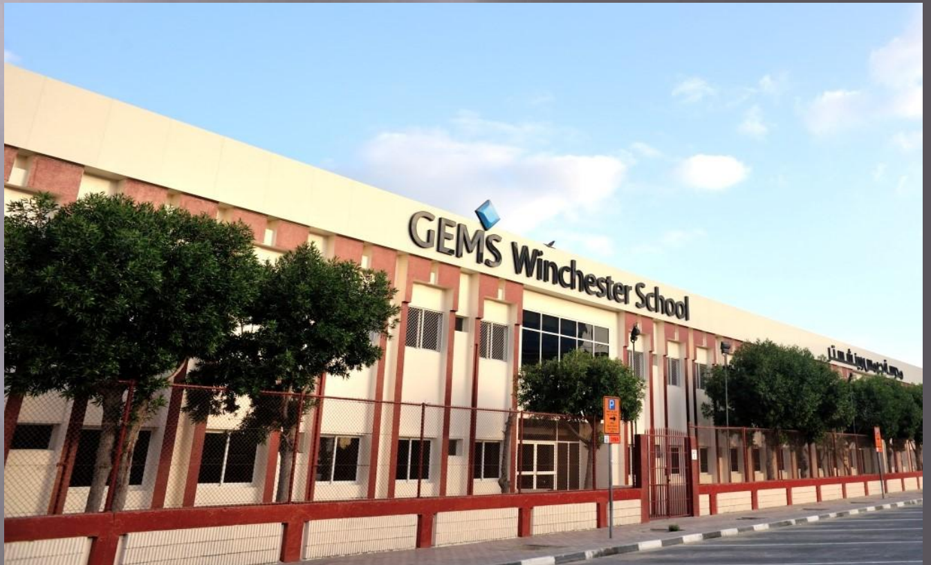
GEMS WINCHESTER SCHOOL PROJECT AT FUJAIRAH
