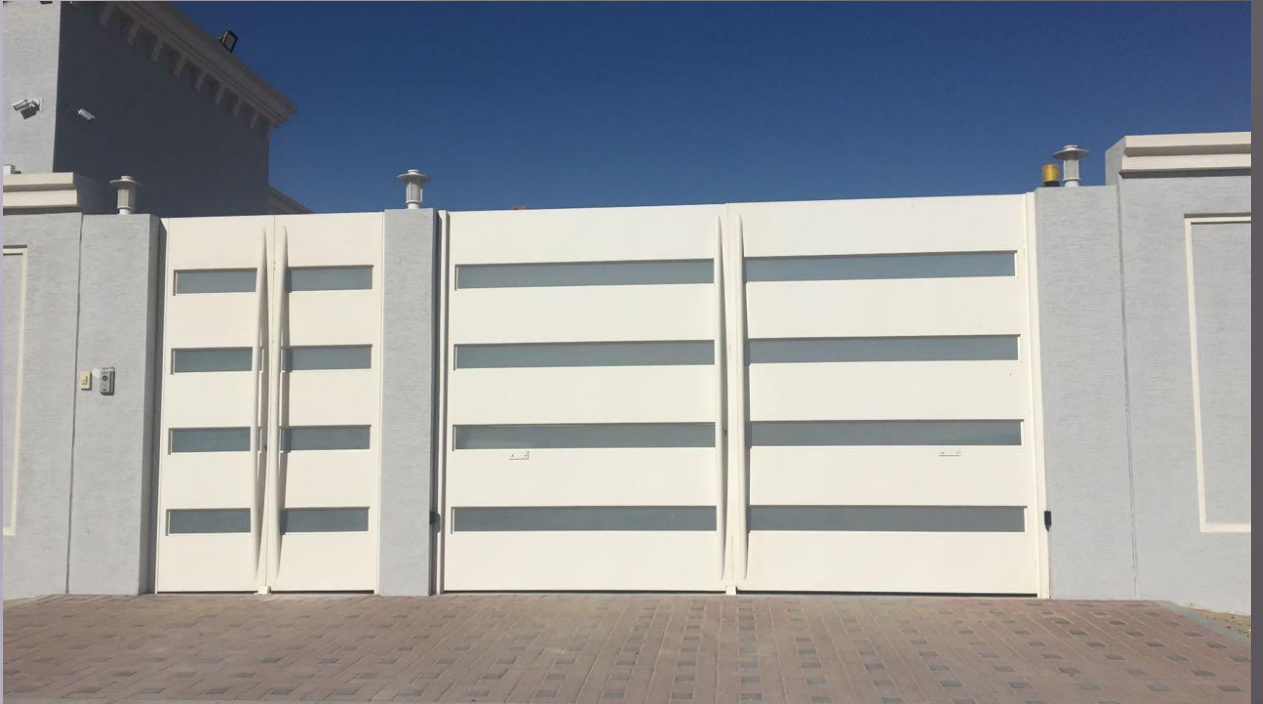
VILLA AT BARSHA
